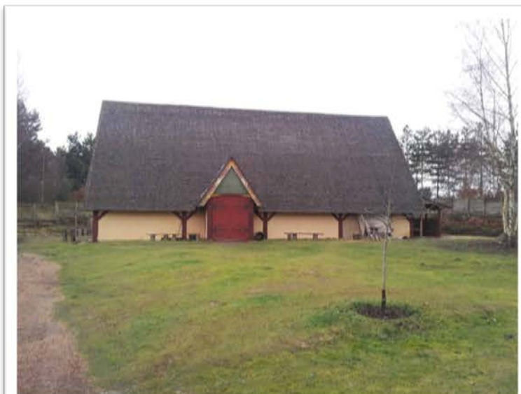
Fig 5 – View of longhall from centre of site.
